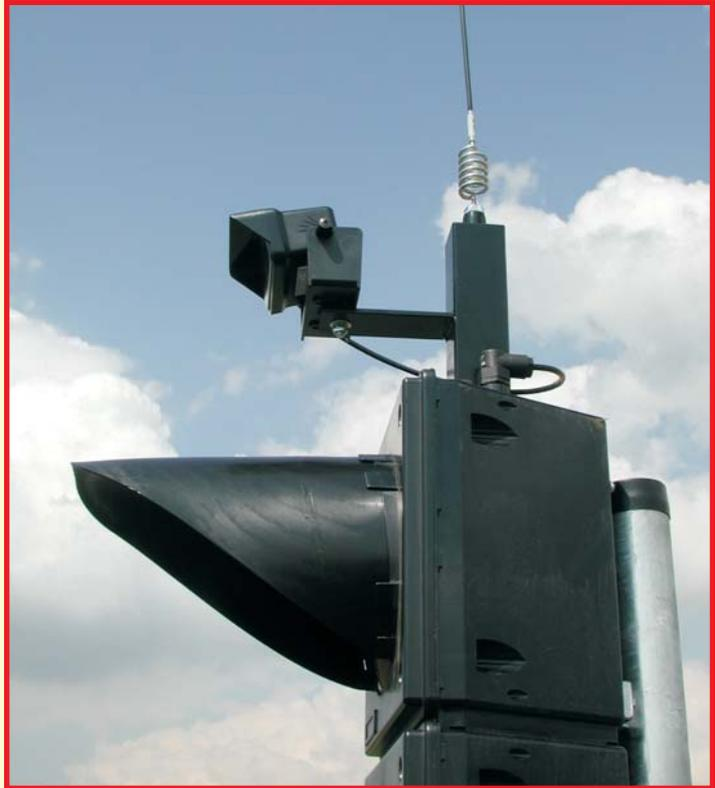
In the interest of trouble-free traffic-dependent control, the signal system is equipped with directional radar detectors as a standard feature for this specific purpose. The road users are informed by an LED in the radar detector that their request has been registered. Reliable all-red mode (green on request) is only possible with directional radar detectors, because these are not susceptible to interference from cross traffic, departing traffic, rain or snow.
